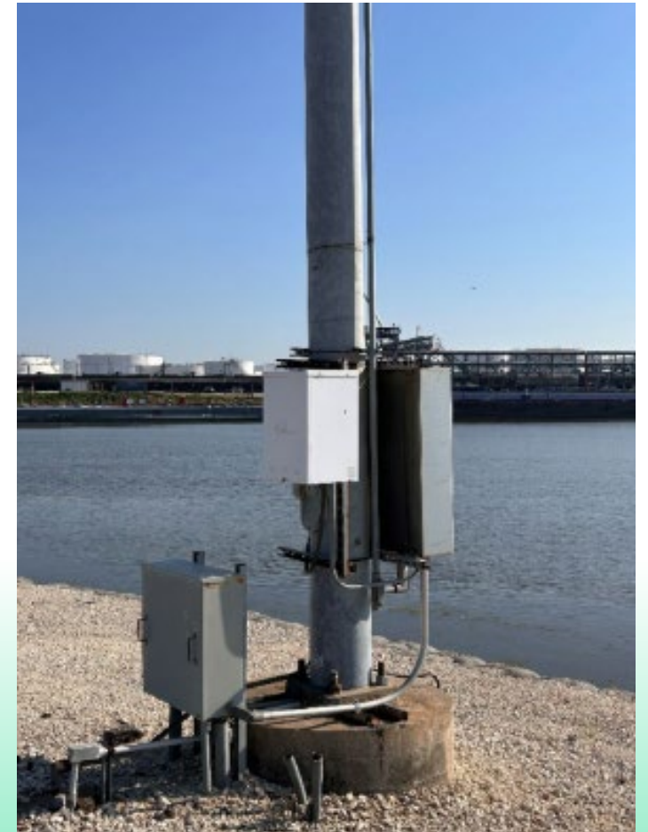
Light Pole Identified for the Installation
